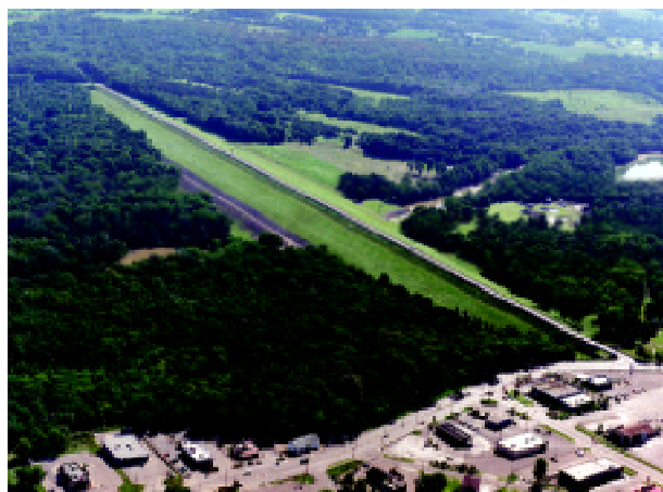
Aerial photograph taken in 1993 shows Englewood Dam as it appears today under U.S. Route 40. Source: Miami Conservancy District
